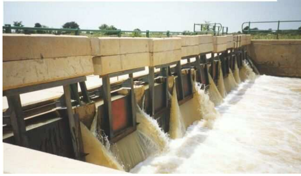
FIGURE 4.43 – Vanne à contrepoids, type Begemann – Hadedgia (Nigéria)
